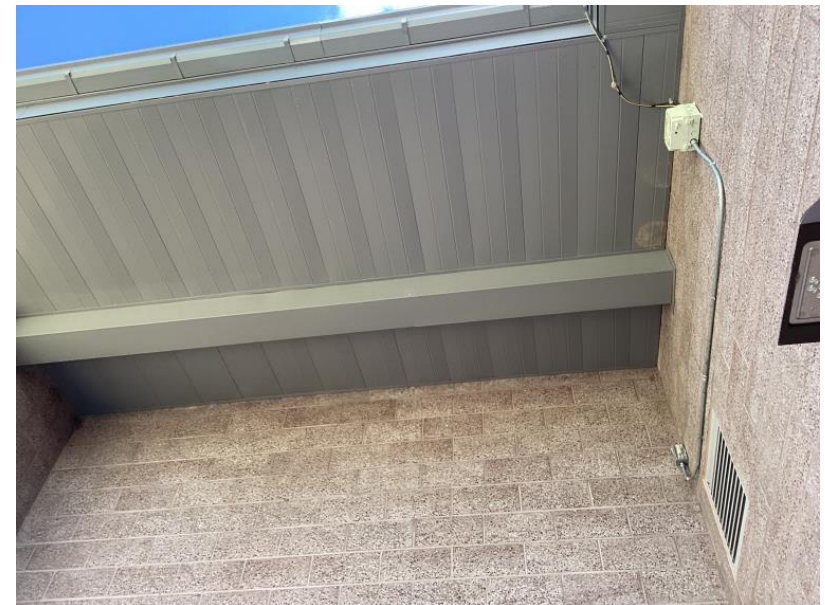
Snow-melt temperature sensor installed under roof overhang.
